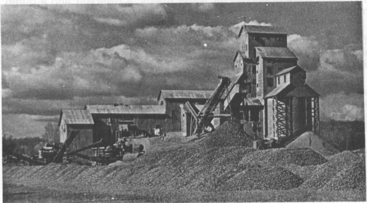
Present day Trap Rock plant.
