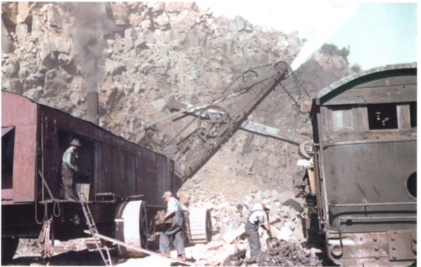
Top: Steam shovels were used to scoop up the large pieces of trap rock and load them into the small dump cars. These ancient machines required a fireman and an operator. Water for the boiler was piped down from a tank high up on the hillside. Bottom: No. 4's train crew is assisting the fireman in hauling coal up to the shovel's boiler while one of the cars is being loaded. All train and shovel movements were signaled with whistles! Both photos, July 18, 1960 —Larry Easton.
