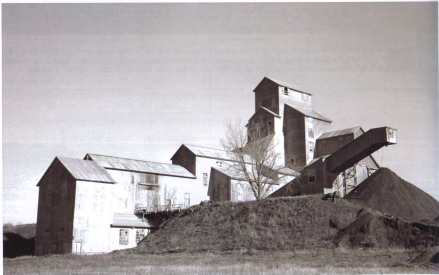
Top: A view from the edge of the quarry. Both shovels are at work filling the cars while the locomotives move the cars into position. The date is July 18, 1960, the author's first visit to Dresser Trap Rock. Bottom: The crusher building was large and multi-levelled. A fire on November 4, 1993 destroyed the building. However, the crusher and storage facilities still operate. This image was captured on Larry's second trip on November 3, 1960 —both photos Larry Easton.
