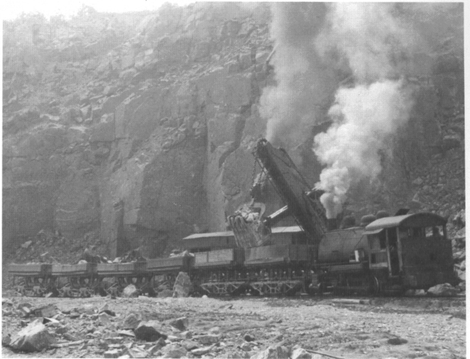
The unique building under construction. Below: The steam shovel fills the dinky cars.
